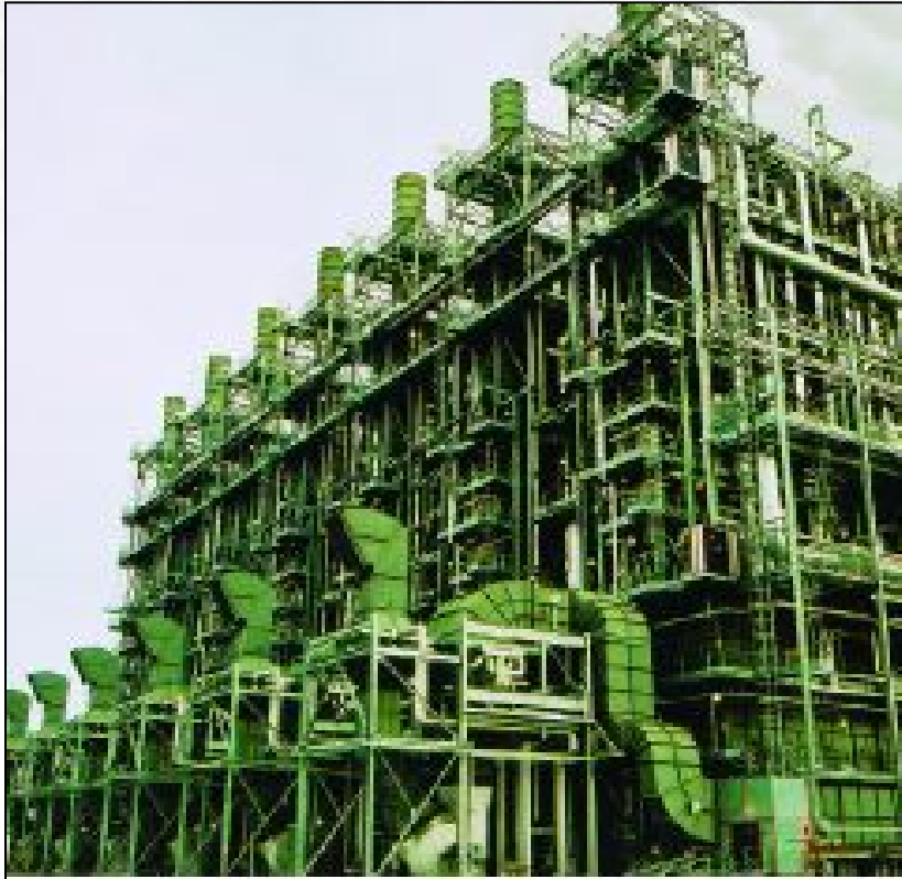
NOVA Chemical cracker; Alberta, Canada
