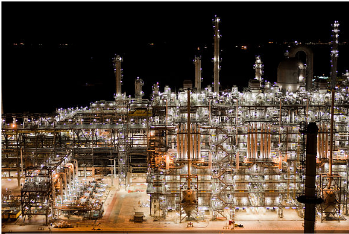
Shell's Singapore Cracker
